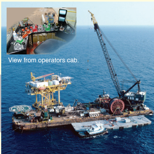
Photo of crane barge working on location for platform upgrading.
