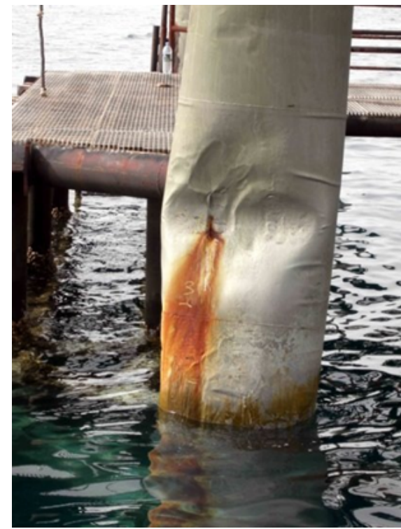
Big dent in the same leg below the leg-pile seam connection
