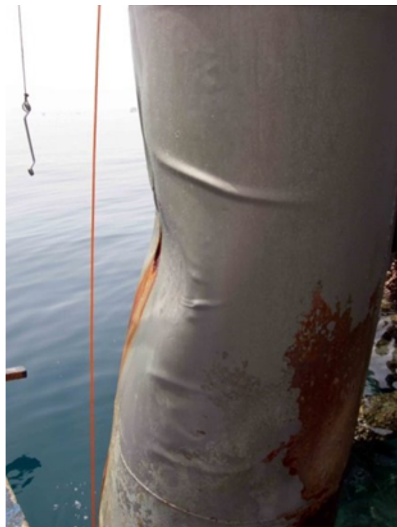
Big dent in the same leg below the leg-pile seam connection
