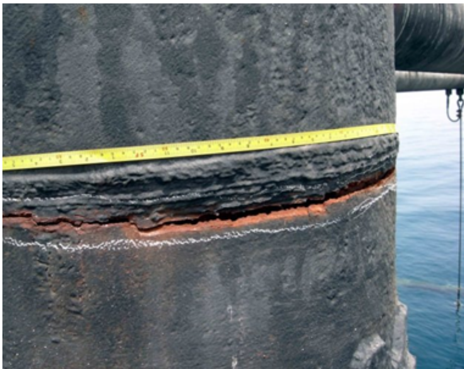
Partial detachment of weld at deck leg to pile connection
